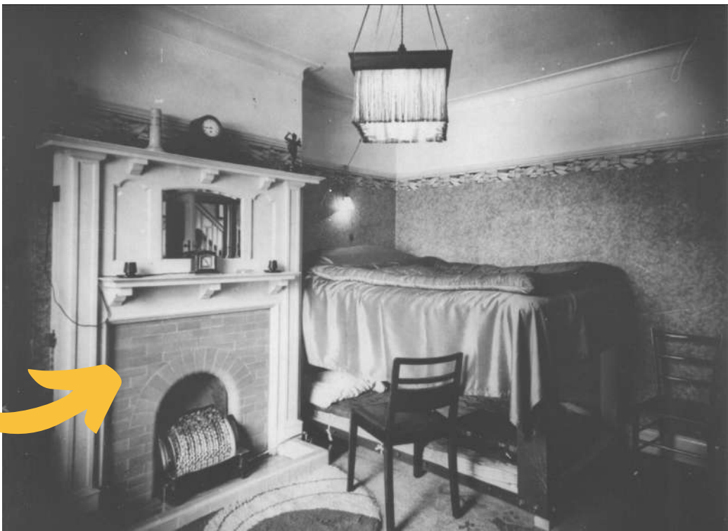
The Morrison Shelter at 19 Boundary Road, Wallington
