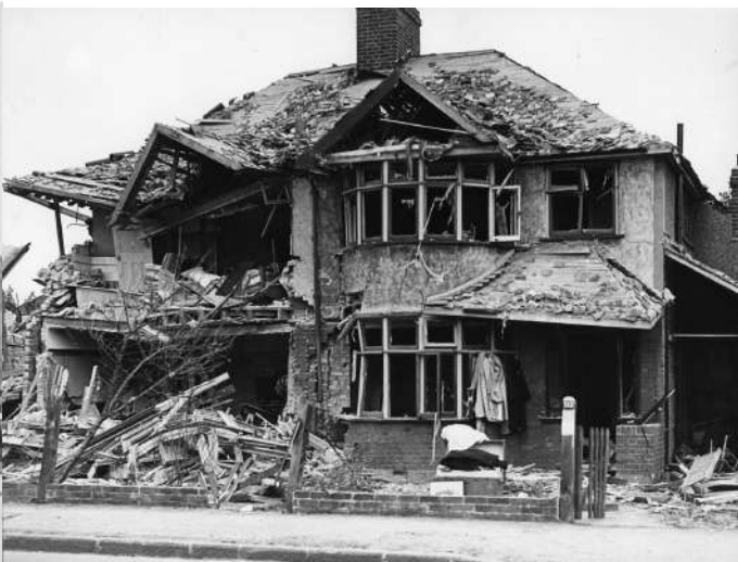
Two bombed houses on Croydon Road, Wallington
